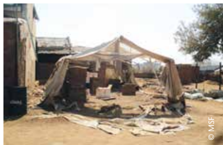
The ruins of the MSF hospital in Frandala, after it was struck by aerial bombing.
